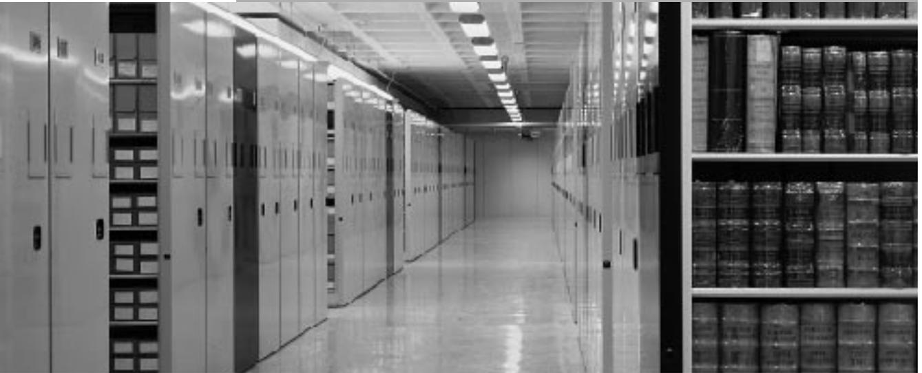
The system compacts almost 2 million cubic feet of storage capacity into an area of 691,572 square feet. The 2,000 carriages roll on more than 80,000 feet (over 15 miles) of rail recessed in the concrete floor.
