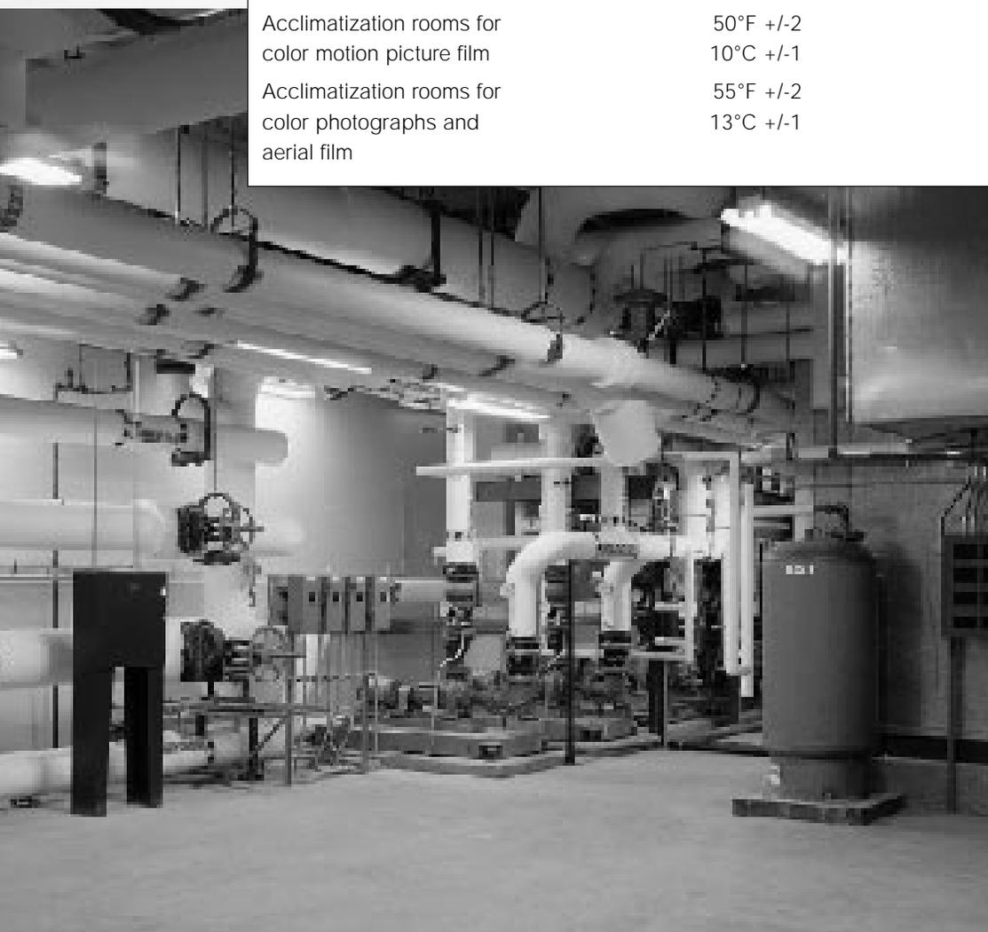
Pressure-reducing stations at various points in the building reduce the steam pressure from 110 pounds per square inch to 15 pounds per square inch for use in heat exchangers, heating coils, and some humidifiers.
