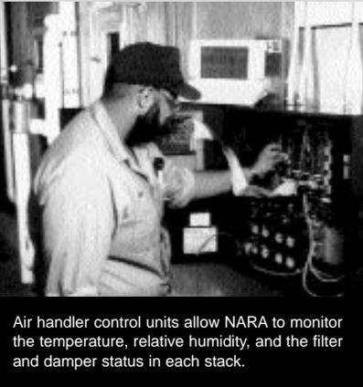
Air handler control units allow NARA to monitor the temperature, relative humidity, and the filter and damper status in each stack.
