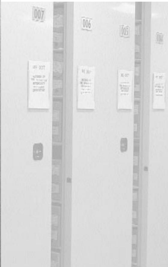
During a fire alarm and at night, the mobile system will leave 4- to 6-inch spaces between the carriages to serve as flues, which reduce the time it takes to put out a fire and the amount of fire damage.
