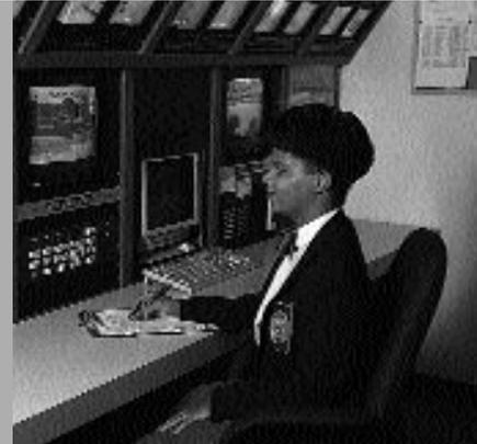
A 24-hour guard service protects the building and staff and monitors the security management system located in the security control room. The console pictured here includes a security computer that monitors intrusion alarms and access, closed-circuit television monitors, a videotape recorder, and a master intercom station.
